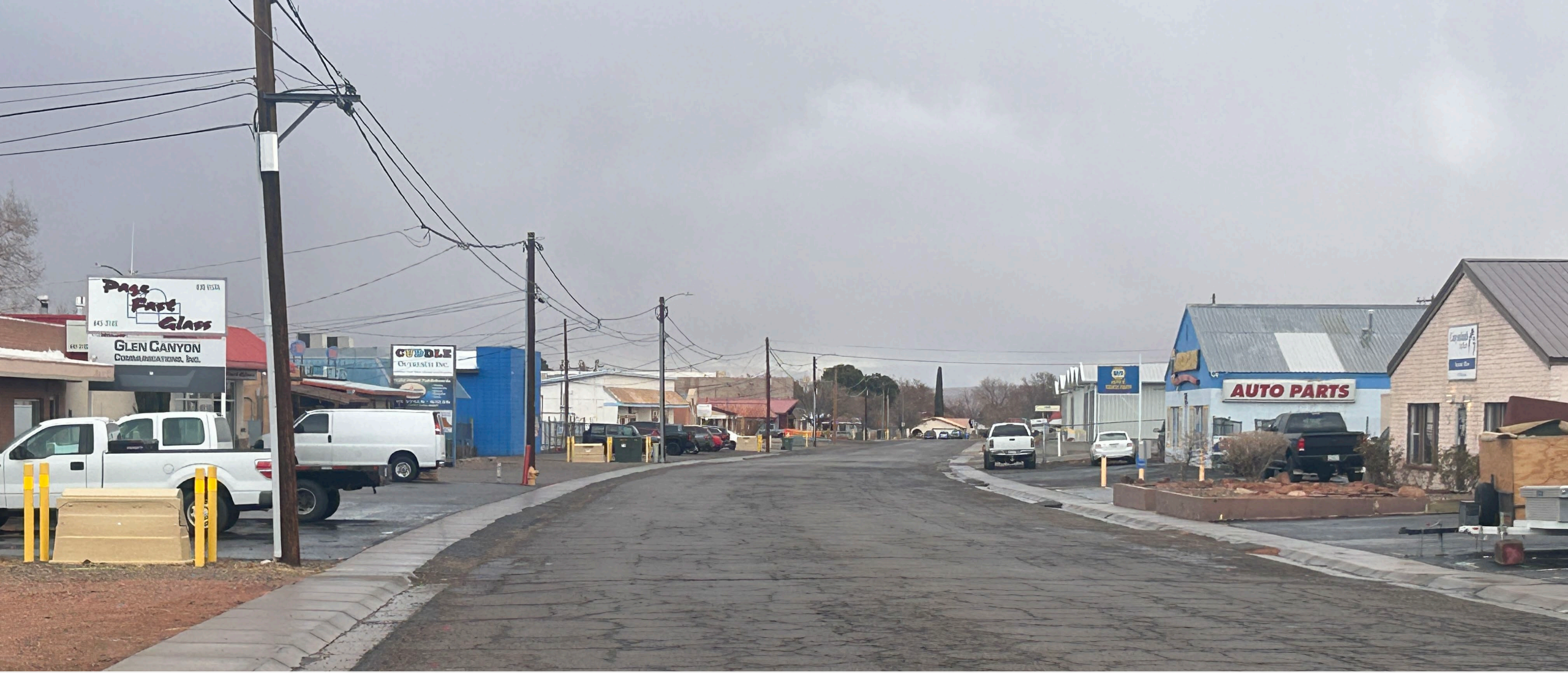
Vista Ave design mill & overlay
