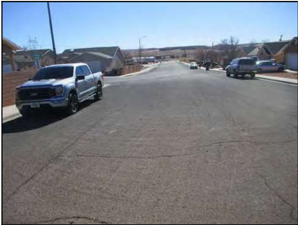
Street view looking south on Newburn Road.
