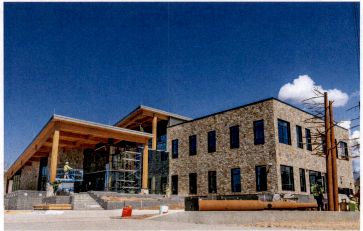
Phase 1 Construction Photo April 24, 2025
