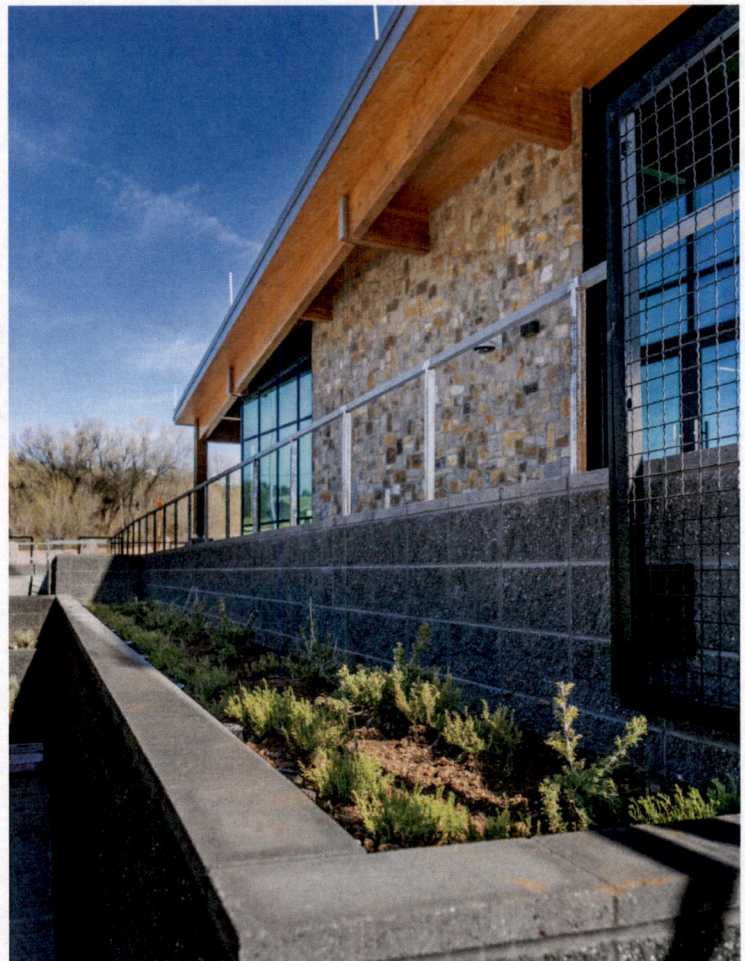
Phase 1 Construction Photo April 24, 2025
