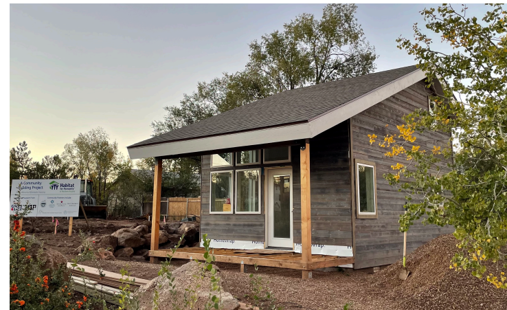
First Starter Home under construction
