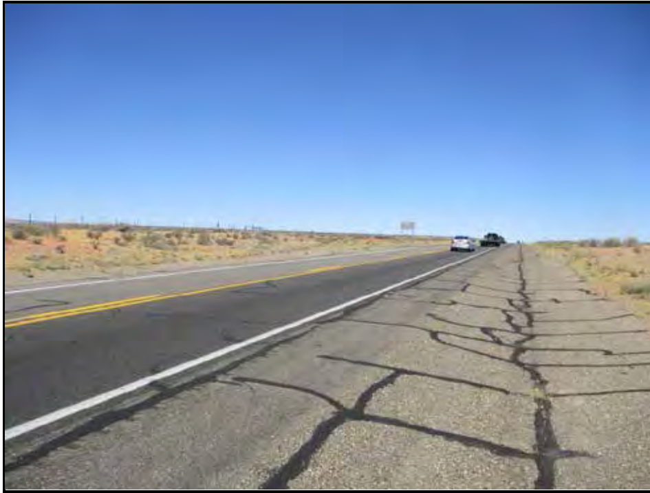
Street view looking northwest on Highway 89.
